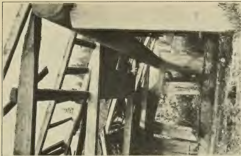
A VIEW OF EAGLE HOUSE "HUT-NES," OLD KASAAN, SHOWING DETAIL OF FRAMEWORK AND THE MECHANICS OF CONSTRUCTION OF A NATIVE HAIDA DWELLING HOUSE
