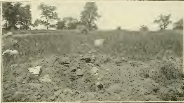
THE BOULDER—AFTER THE BLAST
