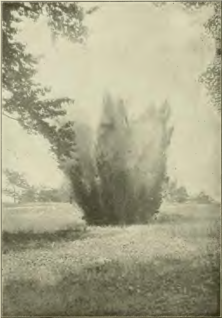
BLASTING A BOULDER
