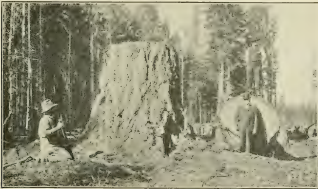
OREGON PINE STUMP—PREPARING FOR THE BLAST
